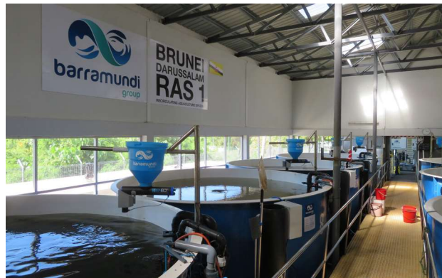
RAS tanks in Brunei are highly automated.
